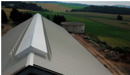
Installation of the steel structure
