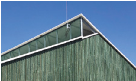
Ridge Vent with Air Flow Control countertop roofs (covering is possible with a roll-up tarpaulin or draught-proof net)
