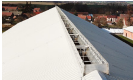
Ridge Vent with Air Flow Control without top arc (for sizes 400–1000 mm)
