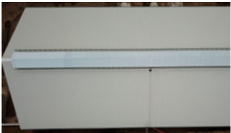
Installation of polycarbonate filling
