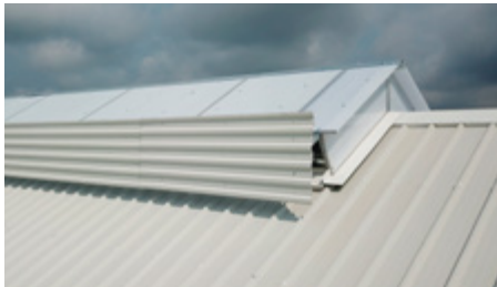
Installation of the side deflector
