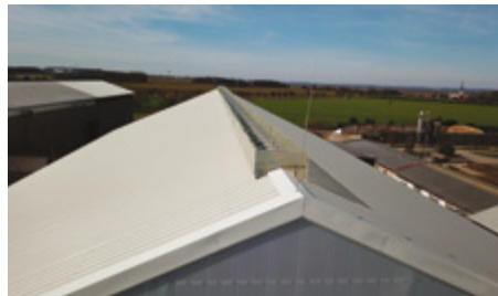
Open Ridge Vent H without Air Flow Control, side view
