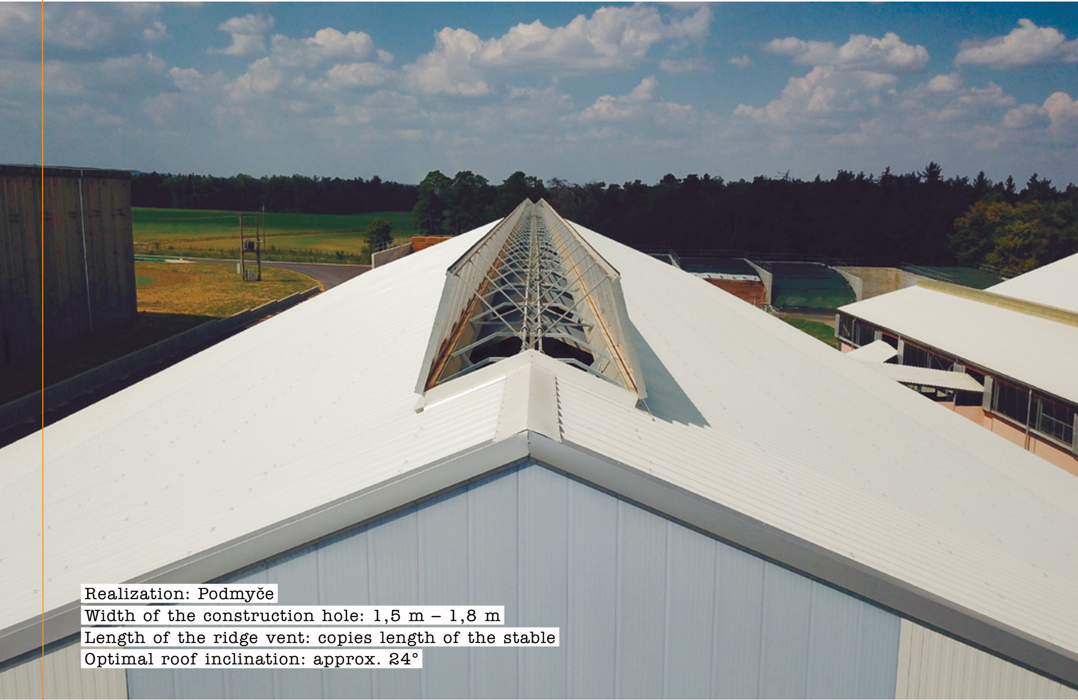
Scheme of Double-Leaf Ridge Vent controlled by an electric drive
