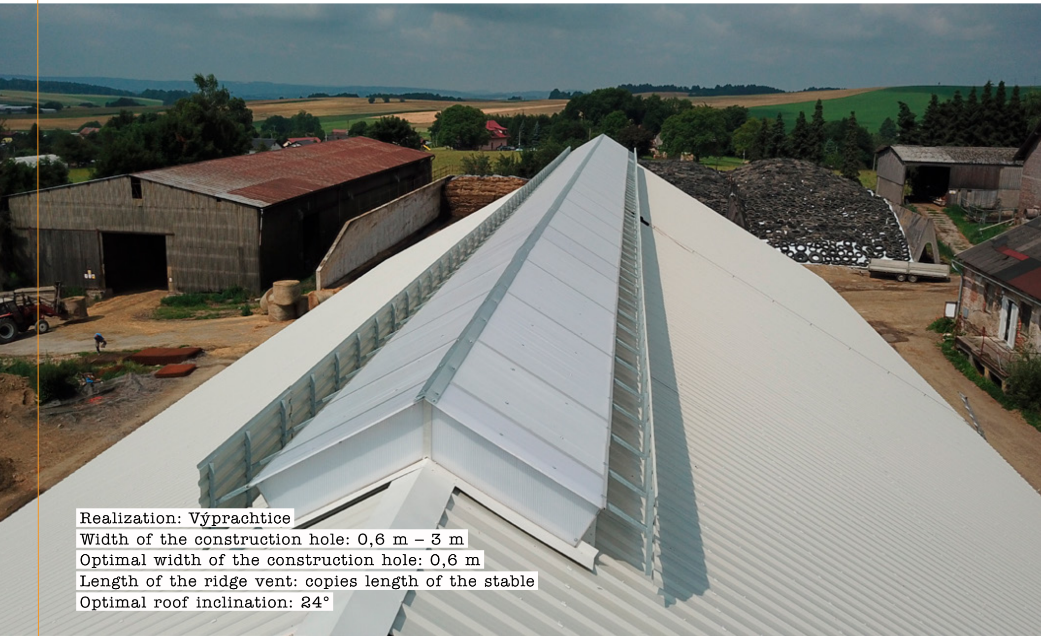
Scheme of Ridge Vent without Air Flow Control – saddle cover
