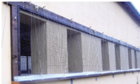
Tarpaulin pulled down on the lower sill
