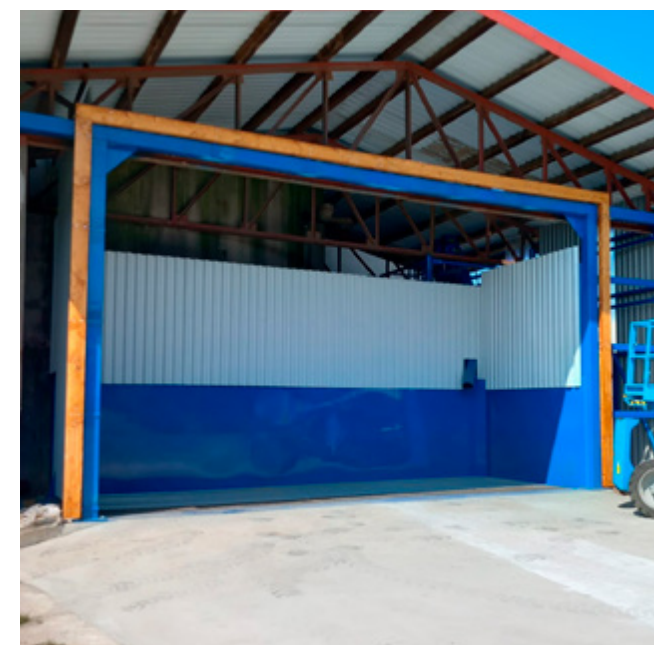
Installation of SVS E Rolling door
