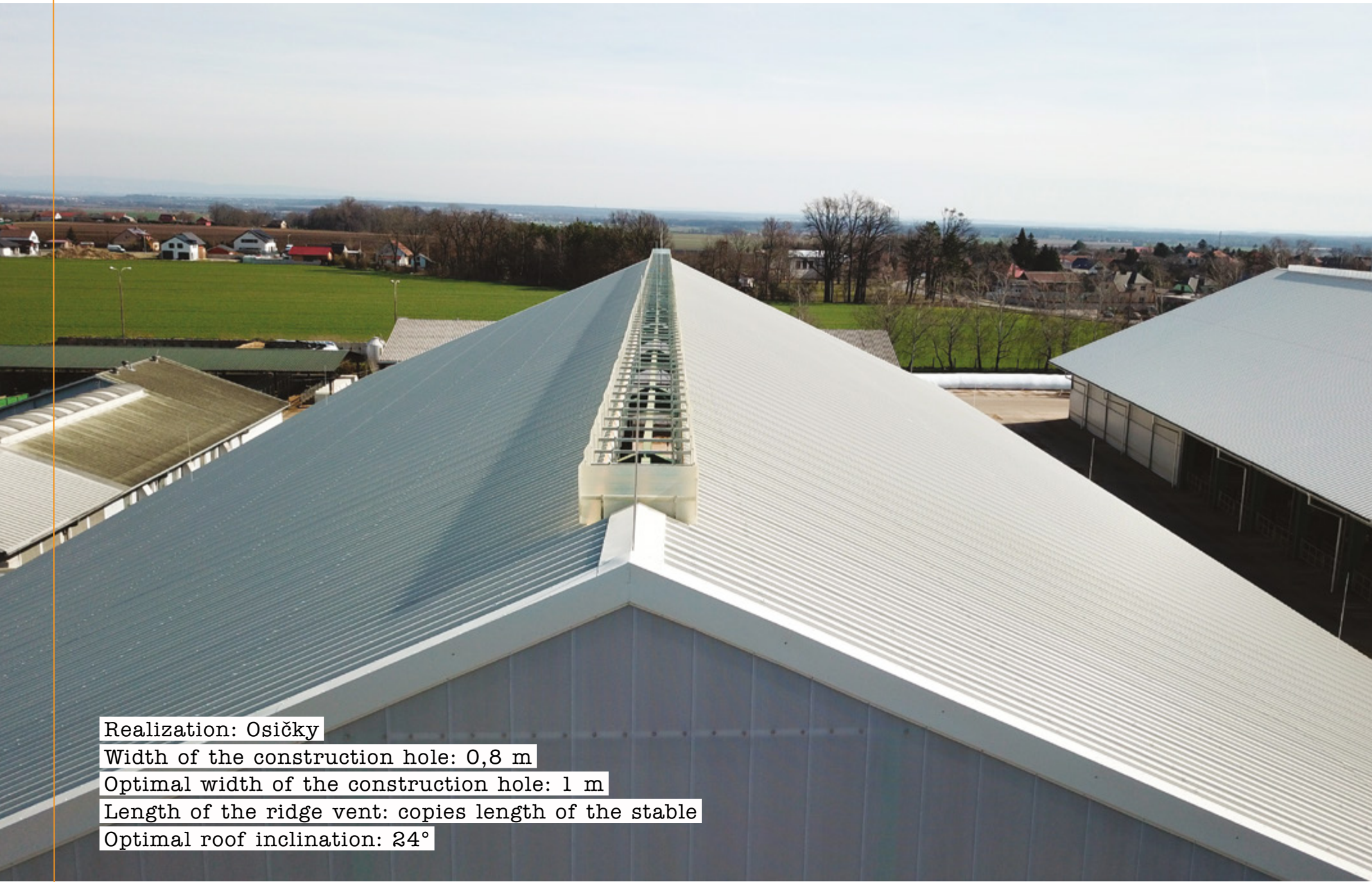
Scheme of a Open Ridge Vent H without Air Flow Control
